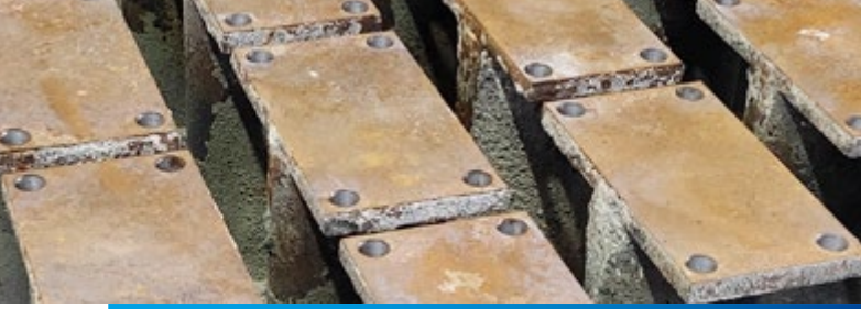
Surface cleaning and overlay welding followed by face milling
