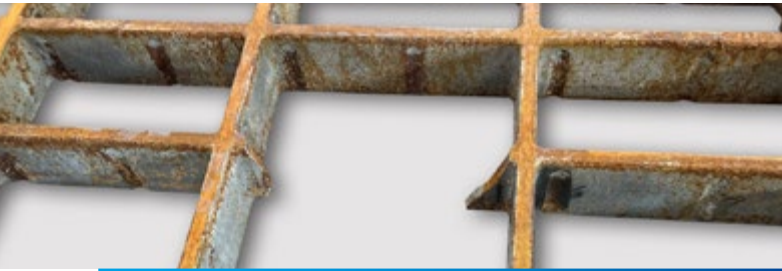
Repair with material replacement
