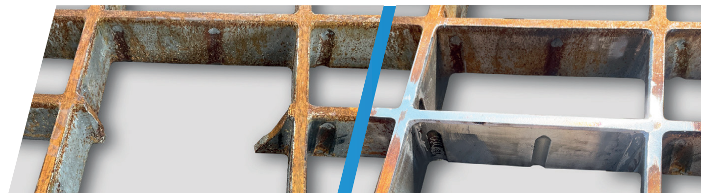
Repair with material replacement
